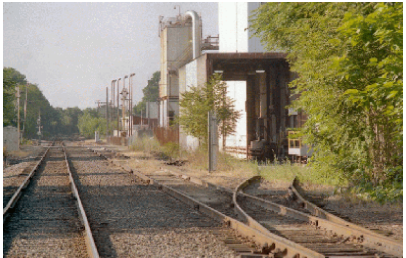
Osram Sylvania, Central Falls. Cars of sand are spotted using the near switch. Light towers in background point to Dean Warehouse doors. {Courtesy Ron Chouinard February 2006}
