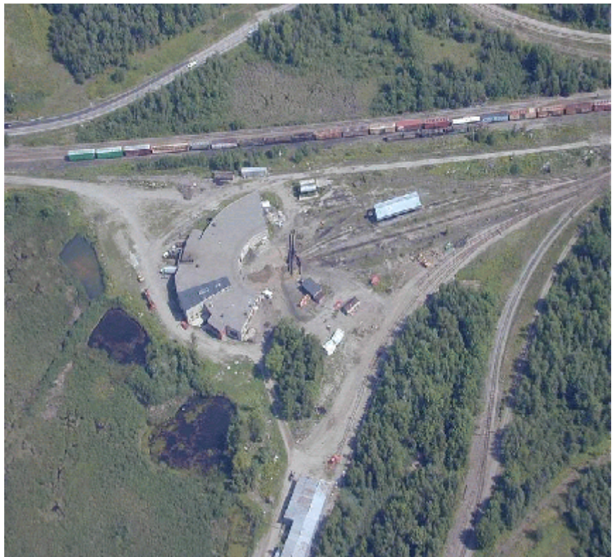
Northern Maine Junction: former Bangor and Aroostook roundhouse , now owned by Bangor Hermon RailYard [see story] and used for storage. The turntable is apparently removed. GRS Freight main runs through photo from left (west) to right (east). {courtesy Kevin Burkholder 20.Aug.05}.
