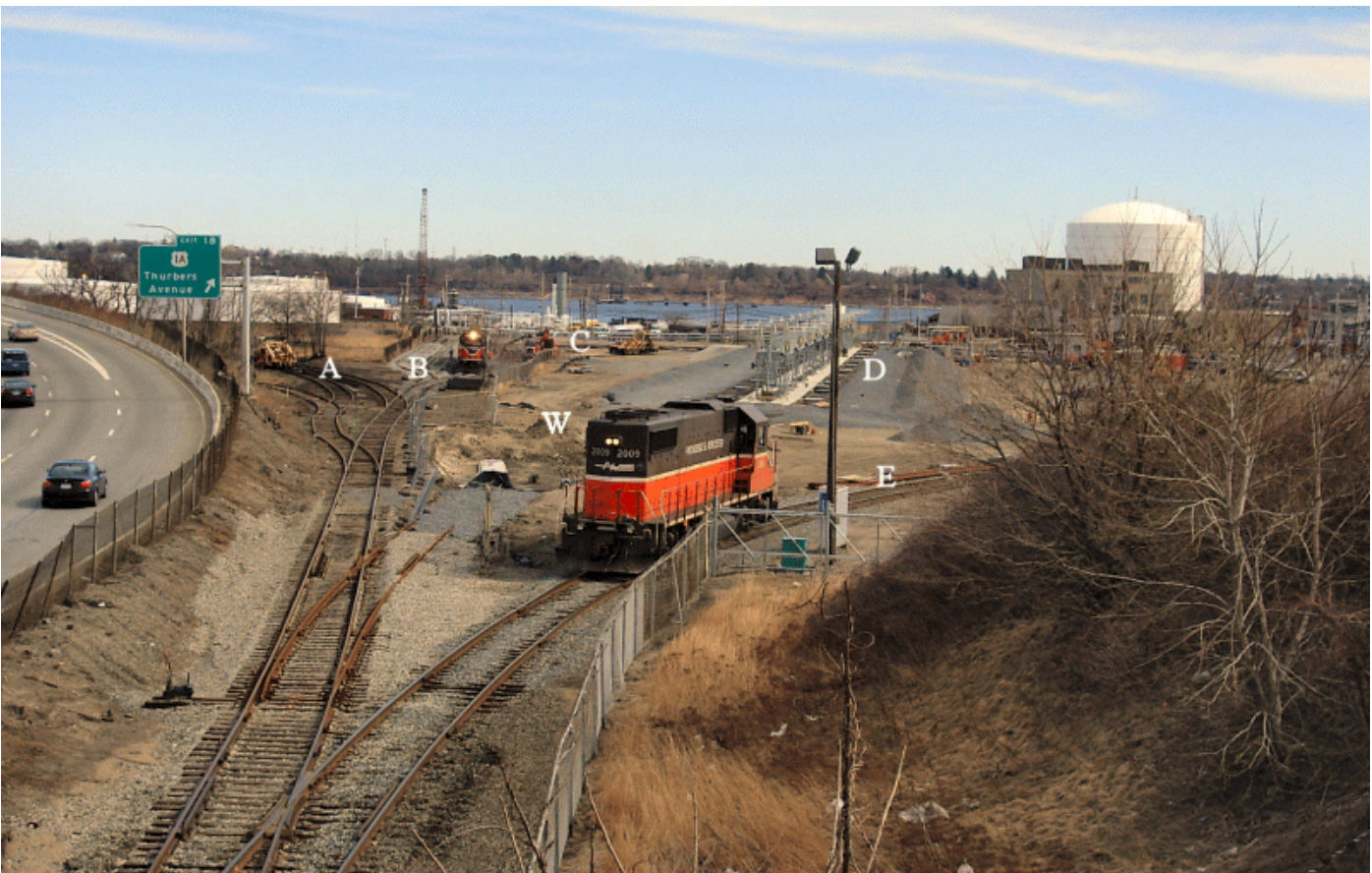
South Providence. (A) Track and spur for Coastal Recycling, not now using rail [see 06#03B]. (B) New three-track South Providence Yard, built by Northern Rail Service and PW [see 06#11B]. (C) Out of service track running across Allens Avenue to the former Providence Gas now New England Gas [see 04#04A]. (D) Ethanol unloading facility with 20 car spots. (E) PW track leading to ProvPort. (W) Site of water main. {photograph and captions courtesy Ron Chouinard}
