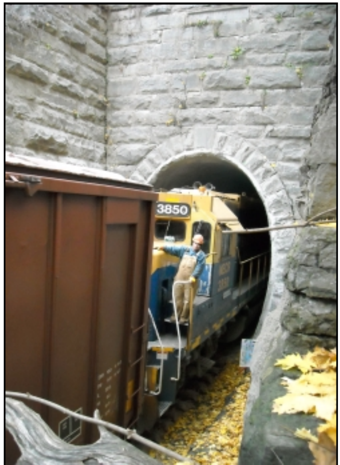
Burlington Vermont tunnel. NECR locomotive showing pre-construction clearance maintained. {courtesy Paul Craven}
